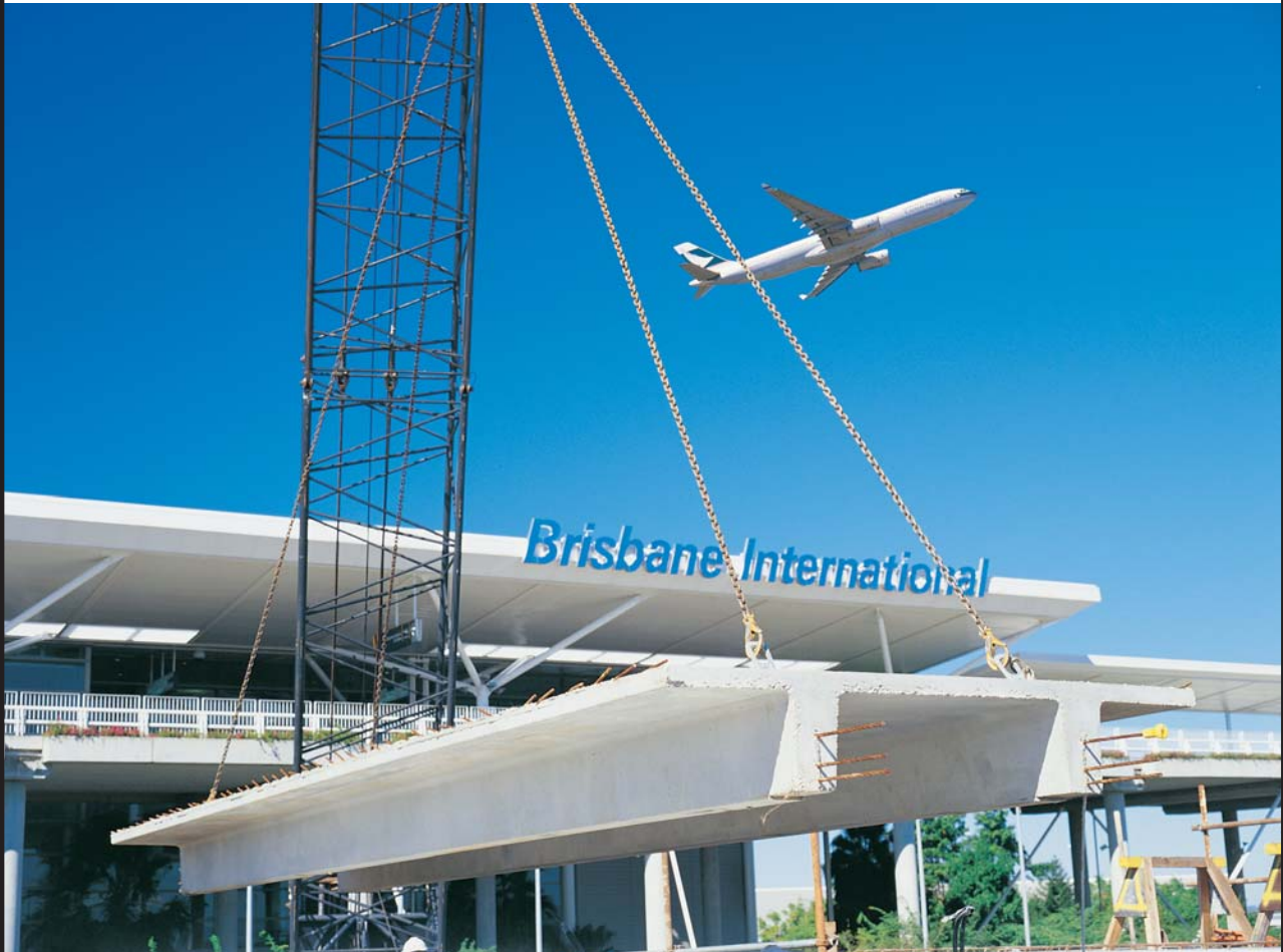
Installation of Maxitee™, Railstation Platforms, International and Domestic Terminals Brisbane Airport
